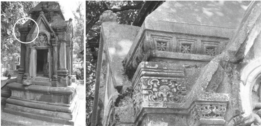
Fig. 8 Earthquake damage to the Payar temple has occurred through lateral displacement of the monolithic roof capstone. At some time in the past nine centuries the roof capstone has shifted \approx 7 cm northward, with no damage to the underlying dressed stone blocks. We attribute the drift of the roof monolith to shaking during earthquakes. A close-up of the offset NW corner of the shifted roof stone is shown right, which, in our opinion, Kak (1933) erroneously diagnoses as a failed attempt to dismantle the temple
