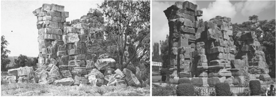
Fig. 11 (Left) Lithograph reproduced from Jones (1885) showing the immediate aftermath of the 1885 earthquake compared to a 2005 photograph from the same angle. (compare with previous Figure). It is possible that Jones took other photos but none were discovered in a search in the Calcutta photographic archives of the Geological Survey of India
