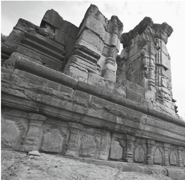
Fig. 17 View from Block 5 (lower foreground) upwards showing west face of the Sugandhesa ruin (much foreshortened by the wide angle lens used in this view). The height of the pillar right is \approx 8 m, and block 5 is believed to have been thrown 0.7 m clear of the ruin from the central pillar, without impacting the lower structure. Note lateral displacement of upper blocks within the columns caused by shaking, and unfinished decoration in the frieze surrounding the basal pedestal. The top surface of this pedestal includes depressions mortised for iron clamps which Kak (1933) noted contained traces of rust. We exposed an iron ingot from Site 6 similar to others that may have been destined to fasten parts of the Sugandhesa ruin now hidden from sight
