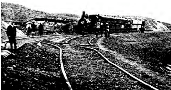
Plate 6 Contraction of the railway line where it crossed the 1892 Chaman fault (from Griesbach 1893). Sinistral fault slip is estimated here to have exceeded 70 cm.
