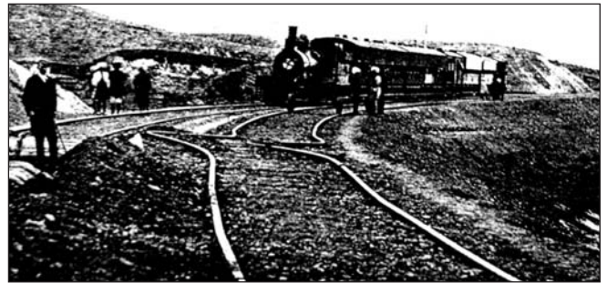
Plate 6 Contraction of the railway line where it crossed the 1892 Chaman fault (from Griesbach 1893). Sinistral fault slip is estimated here to have exceeded 70 cm.
