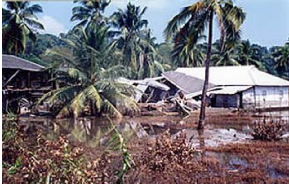
Photo 7: Inundation of the structure in photo 6 and surrounding buildings by the tsunami
