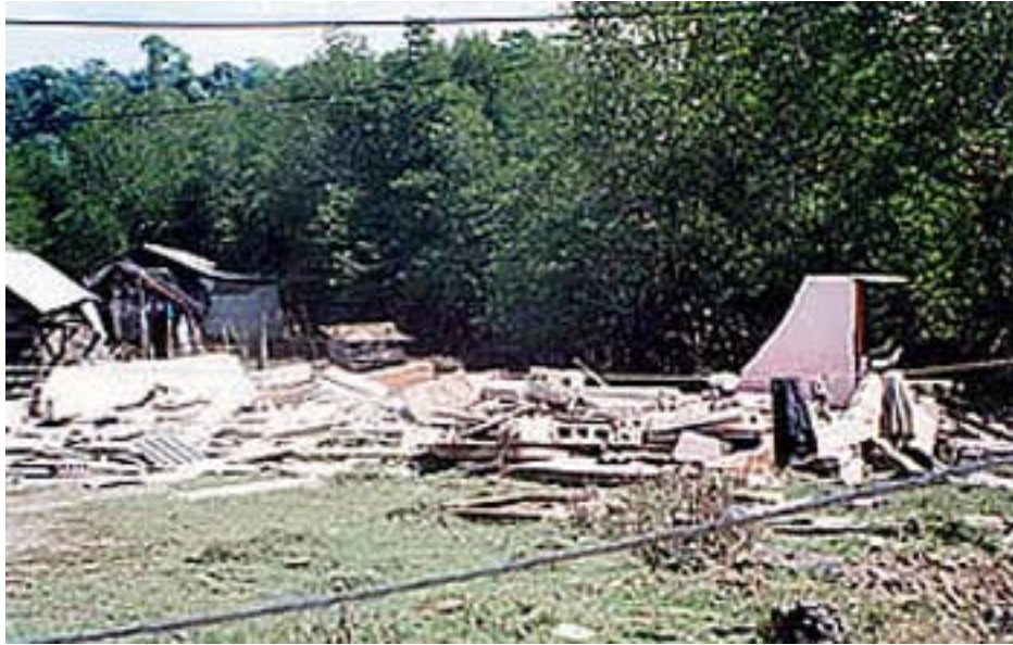
Photo 15: Structures flattened by the tsunami in Wandoor
