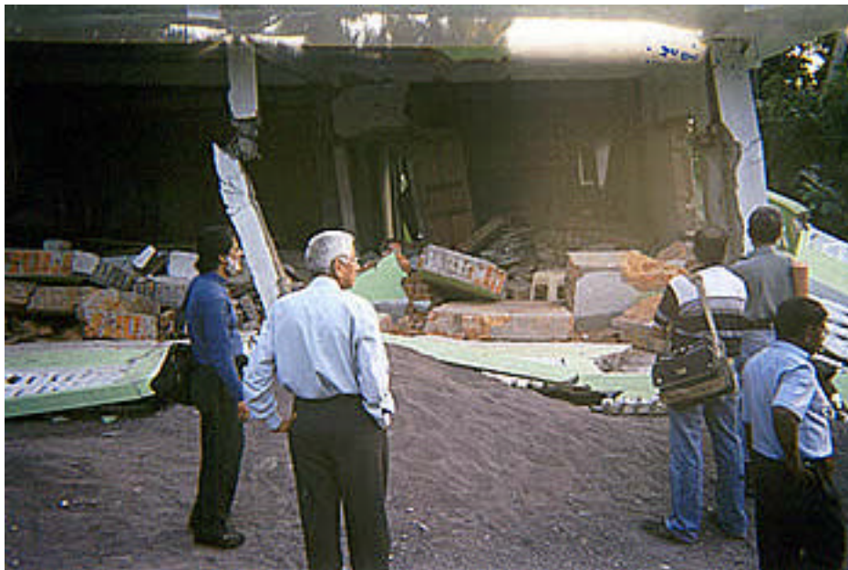
Photo 4: Complete crushing of ground floor due to failure of basecolumn and first floor collapsing to the ground level of a newly constructed building in Bamboo Flat area
