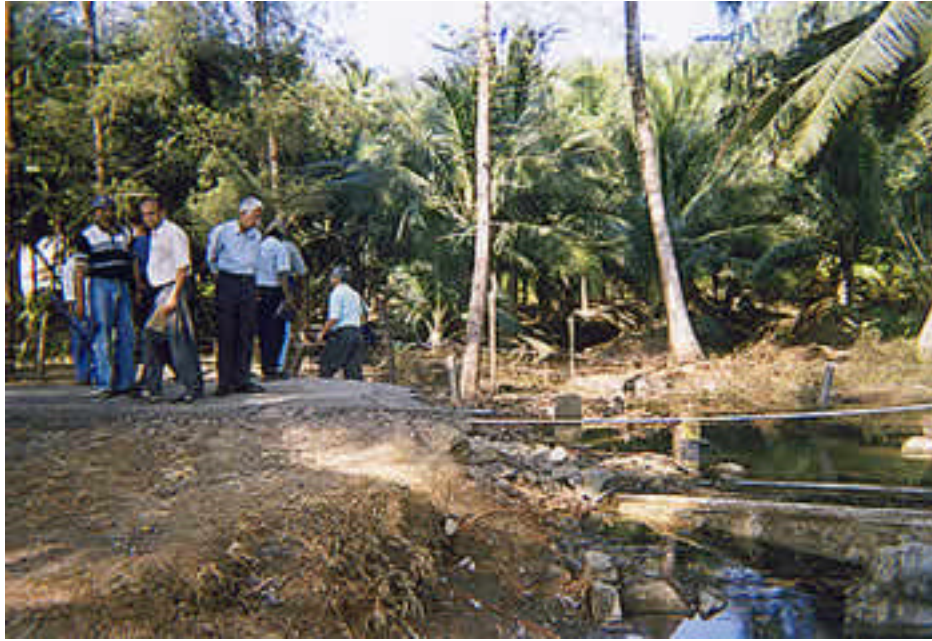
Photo 17: Washing away of a bridge by the tsunami at Corbyn's Cove, Port Blair
