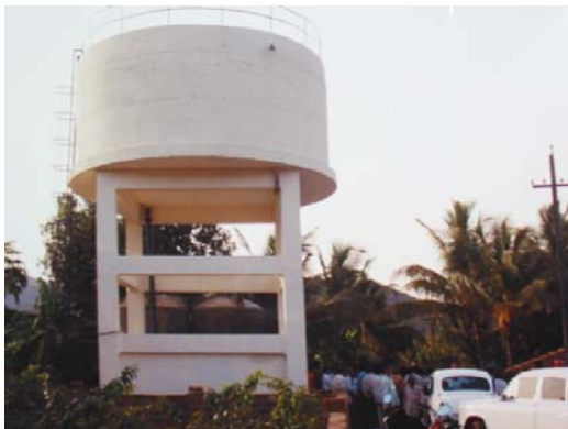
Water Tank Constructed at Mallapur Village
