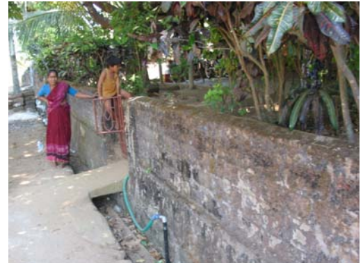
Water pipelines at Mallapur village
