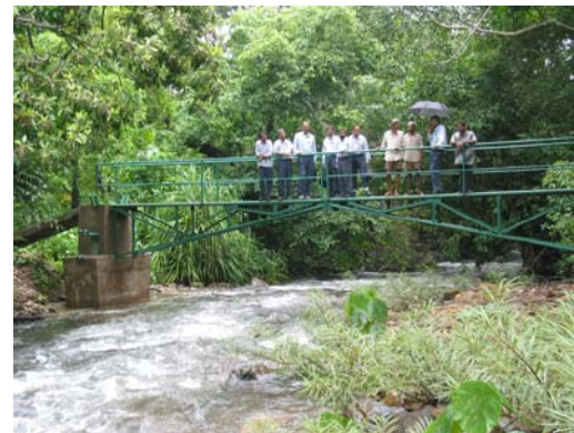
Bridge constructed at Kuchegar Village
