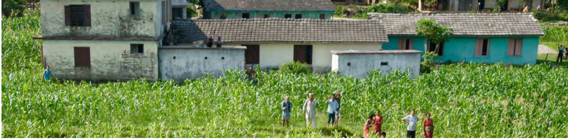
Figure M17. Masonry structures (200 m south of the liquefaction fissure) showed no evidence for damage except of the loss of a few tiles near end gables (Intensity 5-6).
