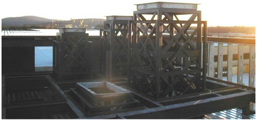
Construction Phase, showing steel vibration isolation cores: siding and hatches now installed
