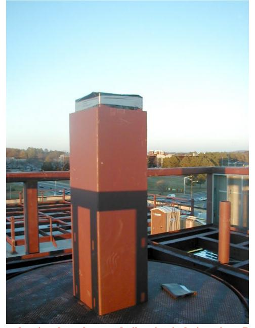
Construction Phase, showing dome base and vibration isolation piers; Dome not yet present
