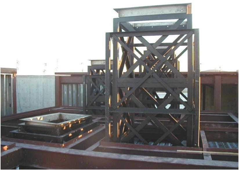
Construction Phase, showing steel vibration isolation cores: siding and hatches now installed
