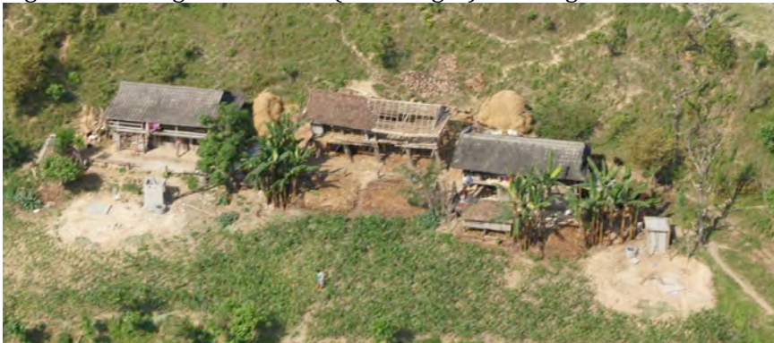
Figure 9 Damage to roof and wooden pillar soft storey misalignment in central building.
