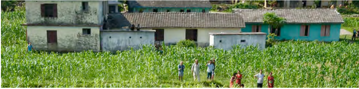
Figure 7. Masonry structures (200 m south of the liquefaction fissure) showed no evidence for damage except of the loss of a few tiles near end gables (Intensity 5-6).
