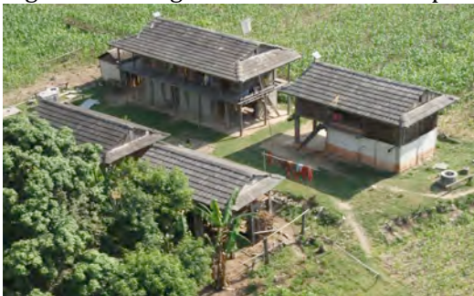
Figure 10 No damage to masonry ground floor or wooden superstructure and roof.
