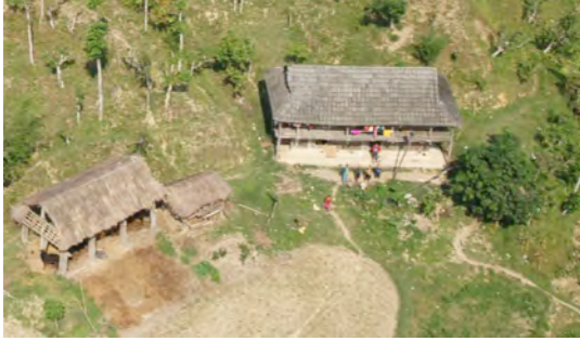
Figure 11 No evident damage to lightweight soft story barn. Possible loss of end-porch roof cover lower left.
