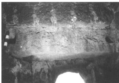
Figure 12. Grapnel stone anchors noticed as lintel on the arches of the parapet wall of the second fortification of Vijaydurg Fort (Photo: S. N. Bandodkar). Scale in 5 cm units.
